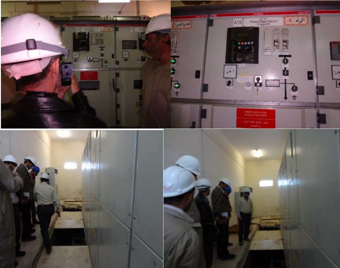
(Switch gear upgrade)
