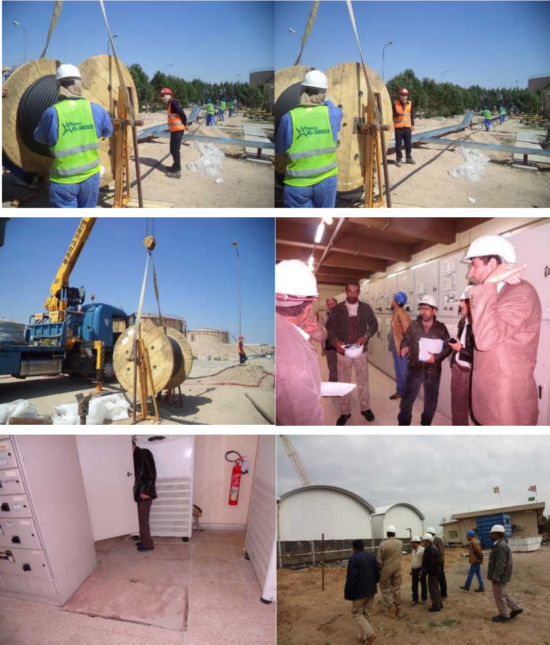
(Cable laying with Galvanized for fire and gas PLC systems)
