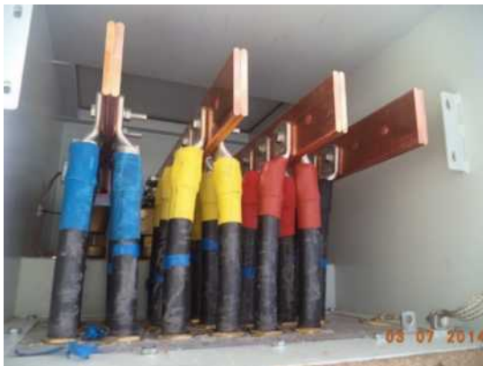
(Power cable installation of Zubair Mushrif generators set)
