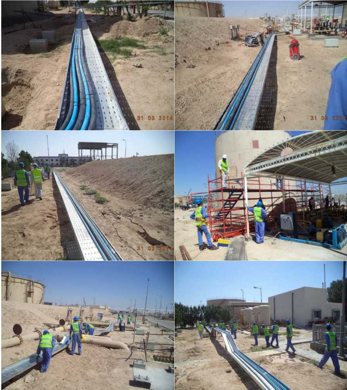
(Cable laying with Galvanized for fire and gas PLC systems)
