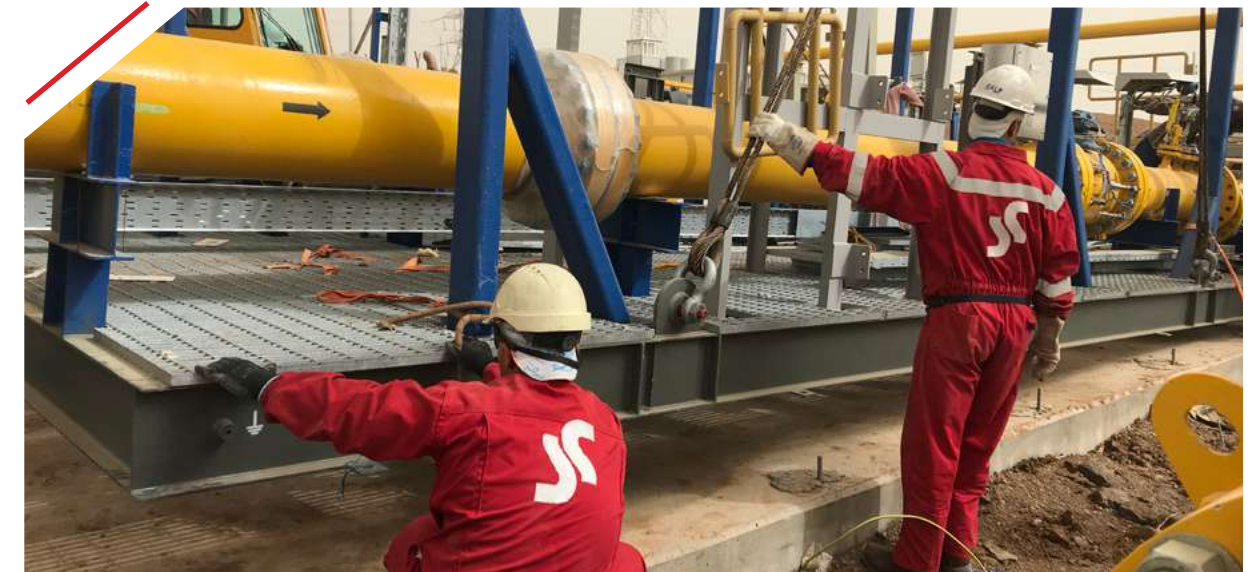
On the tie-in point, SALP built the Gas Metering and Pig Launching station in Chemchemical at Dana Gas tie-in station.
