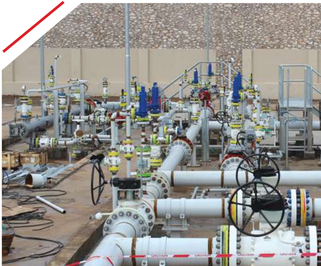
Intermediate Pigging and Pressure Station – Atrush
