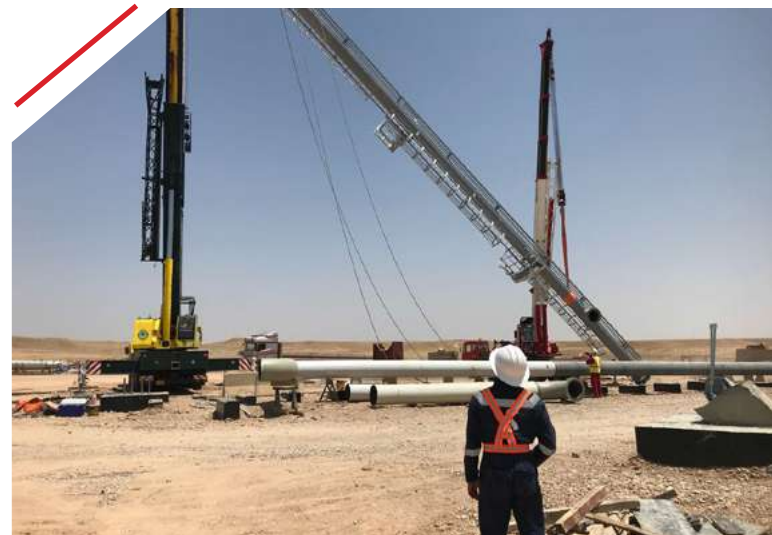
HP flare installation in GPNME CPF brown field project.
